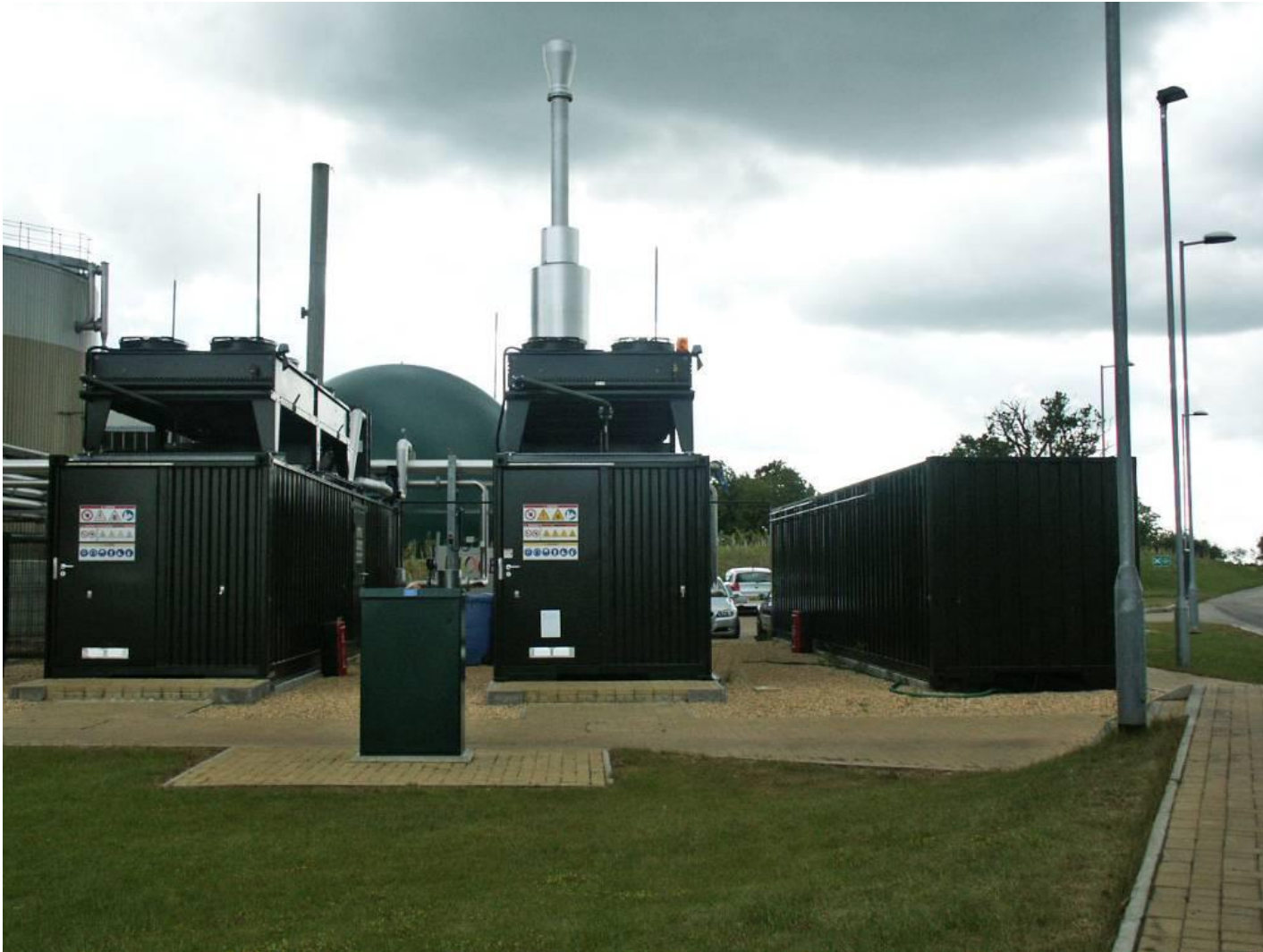
Combined Heat & Power (CHP) units
